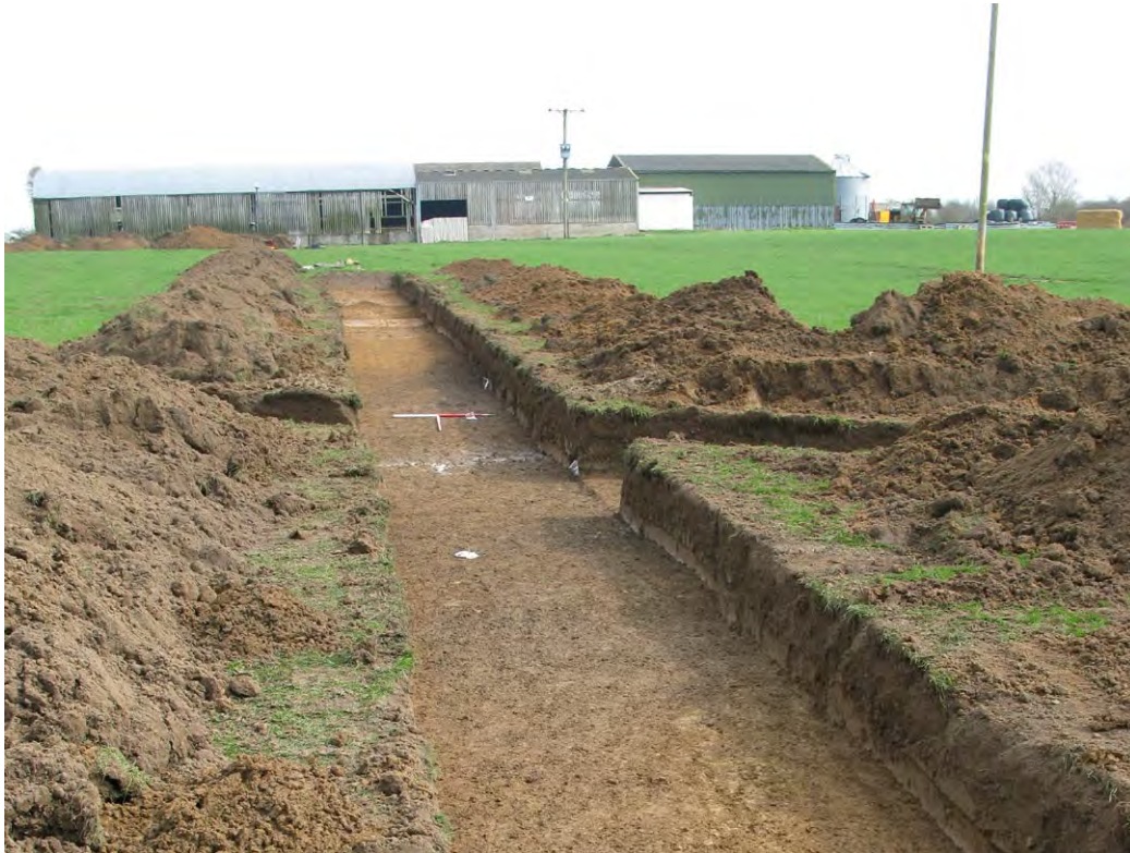
Fig. 1.11.3a - Shot of Ditch 190106/15 (pre-excitation) in Trench 1901, from the W
