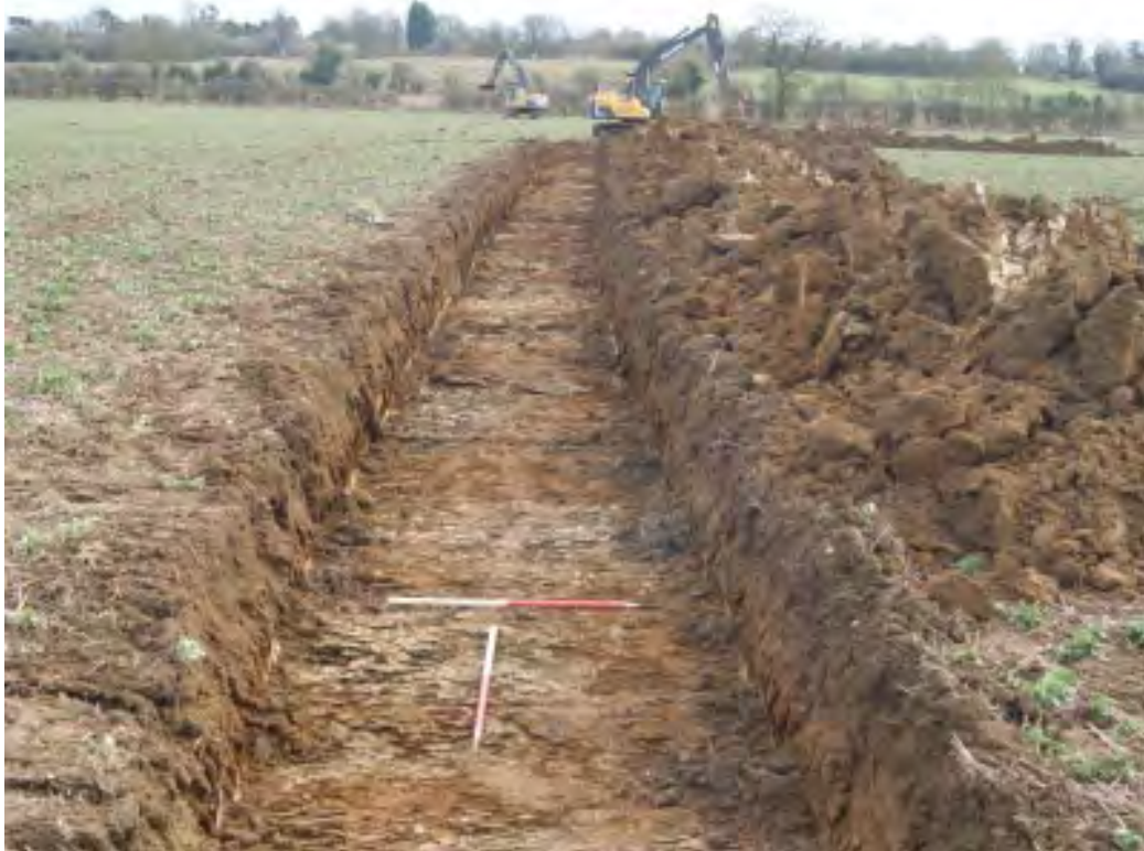
Fig. 1.2.3f - General view of Trench 4213, from the W
