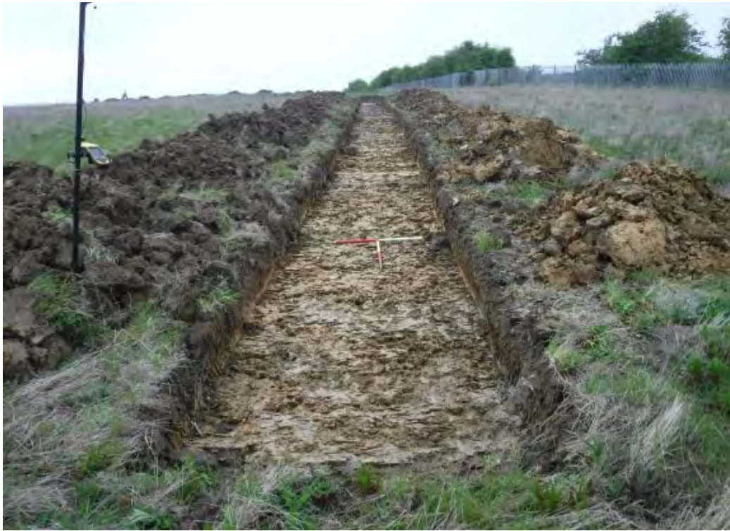
Fig. 1.12.3g - General view of Trench 3906, from the S
